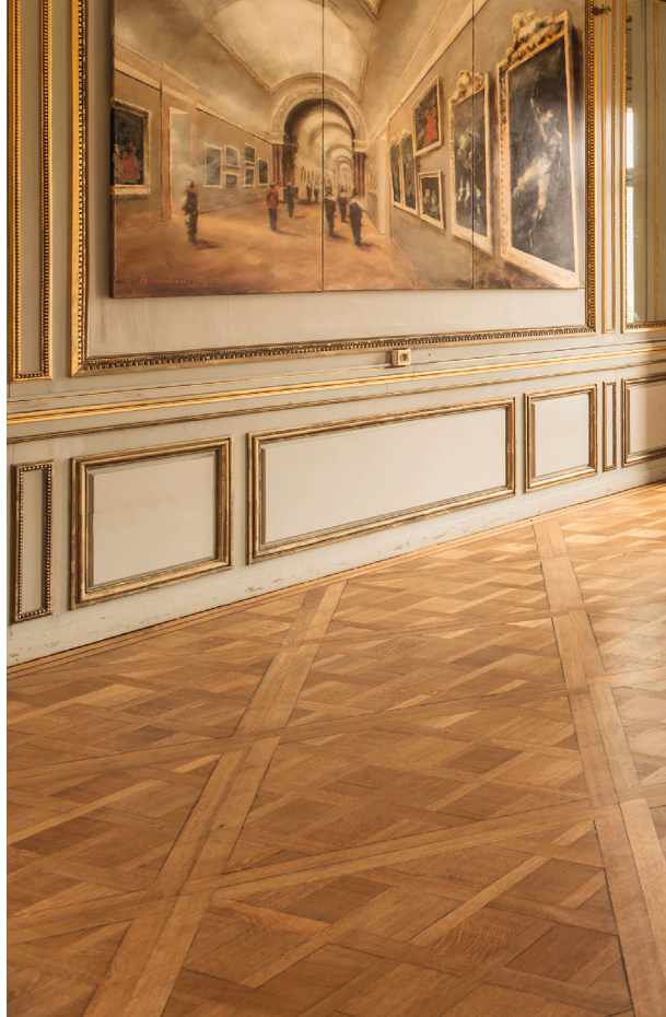
2 final coats for commercial work.
